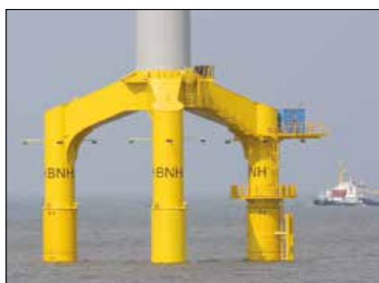
▲ Offshore wind turbines levelling: Enerpac's synchronous lifting system was the solution for levelling support cross pieces on 80 wind turbines.
