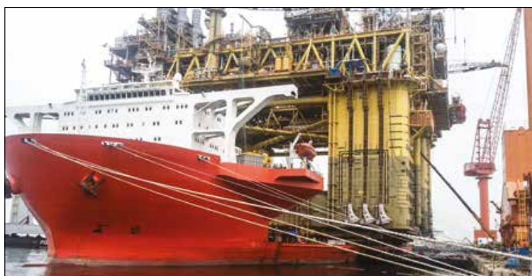
▲ The superlifting and launch of a 43,000-ton floating oil production system in Malaysia for the Gumusut-Kakap offshore field has set high benchmarks for safety through its use of sophisticated EVO-Series synchronous hydraulics to lift, balance, weigh and smoothly launch massive resource structures.
