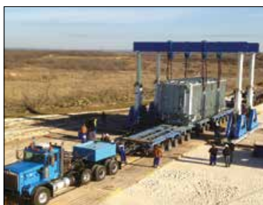
Transformer Installation with a Hydraulic Gantry
