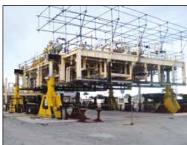
Assembling an Offshore Platform Oil Rig Module
