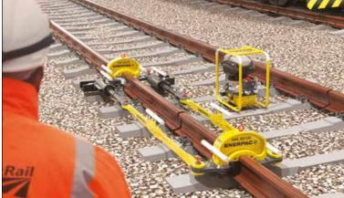
Special Energac ZC3-Series Cordless . Hydraulic Pump used for rail stressing applications (page 190).
