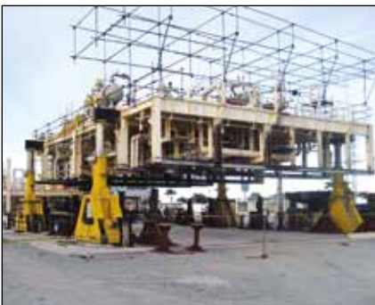
Assembling an Offshore Platform Oil Rig Module
