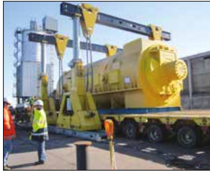
Turbine Lift and Load-in at Shipping Port
