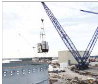
▼ Rigging engineers used the SyncHoist system to precisely monitor and adjust each lifting point independently, or together in a synchronized manner to position the 1140 ton nuclear plant module.
